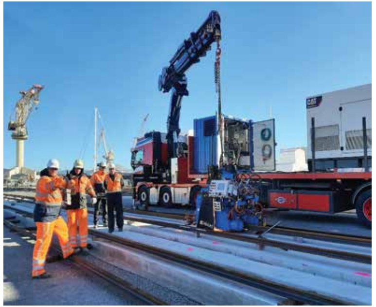
Figure 2: Holland G-Head welding crane rail
