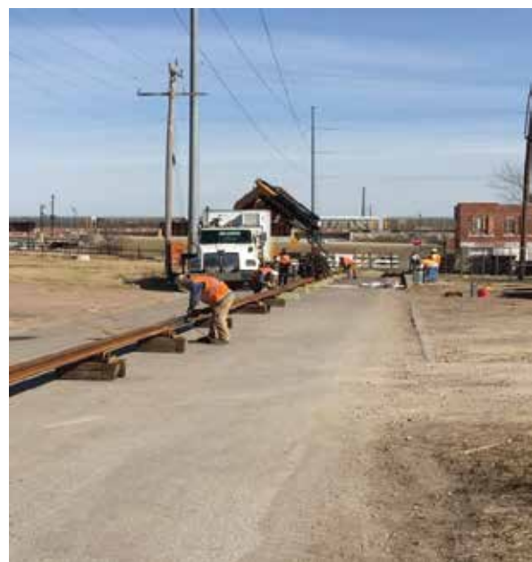
Figure 1: Oklahoma Streetcar Project welding 51R1 rail from Voestalpine
